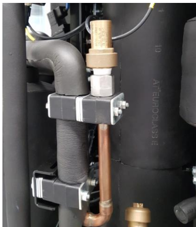
Figure 32: Pressure relief valve on high pressure side
