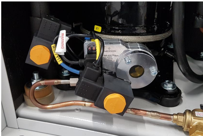
Figure 36: OM5 TraxOil mounted on the compressor
