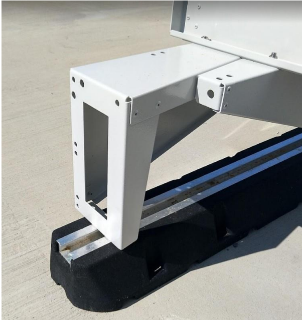
Figure 50: Unit mounted on concrete slab with anti-vibration pads
