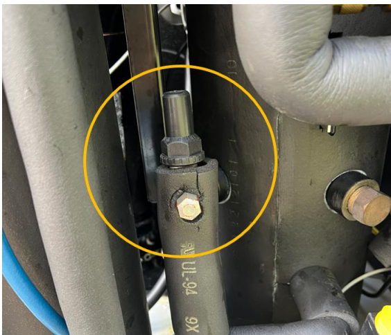
Figure 45: Close up of shut-off valve after liquid receiver
