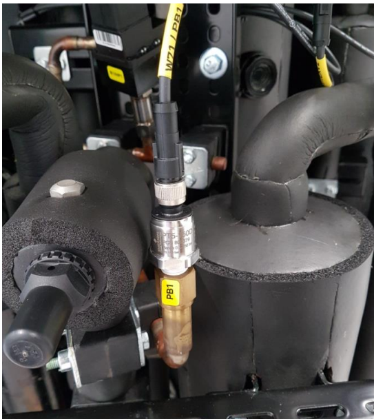
Figure 34: Low side pressure transmitter
